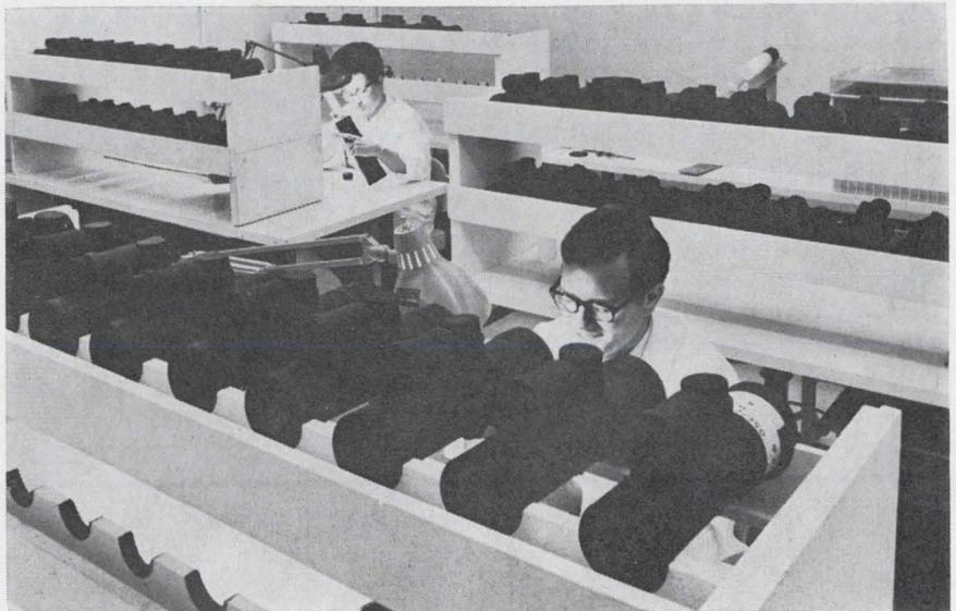
**On the line.** Technicians assemble Starlight night-vision scopes for the Army at Electro-Optical Systems in California.
