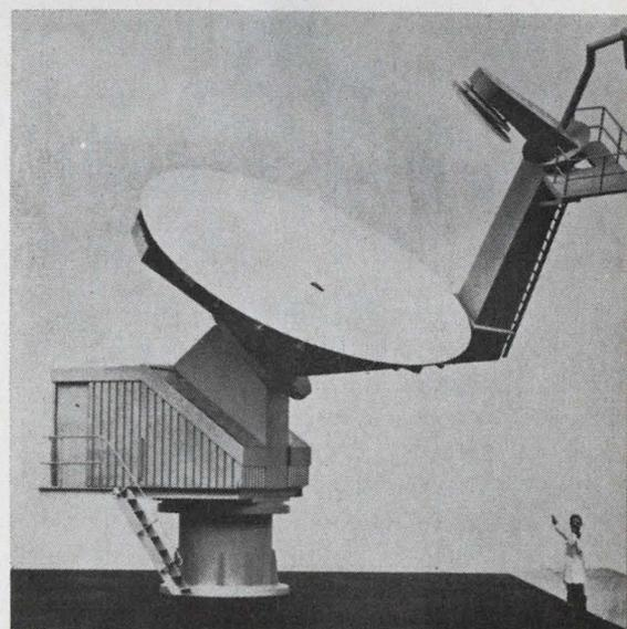
**It swings.** Off-center layout for subreflector betters noise characteristics and gain of small Cassegrain antenna.
