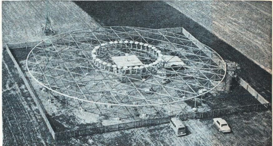
**Antenna carousel** for doppler VOR system at Ruedesheim, Germany, projects above mesh-covered support frame 130 feet in diameter. Azimuth-variable signal is switched around antenna ring electronically.
