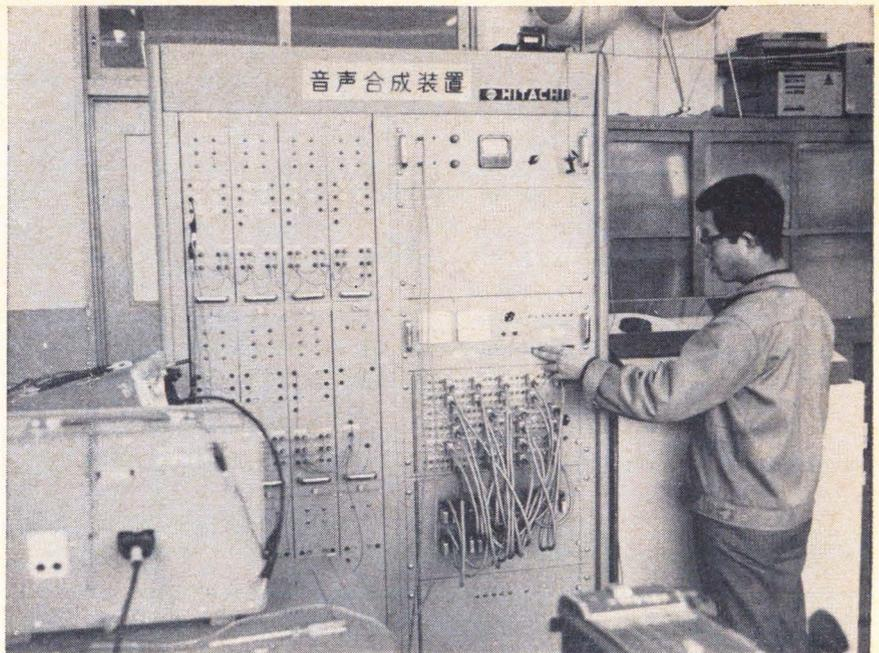
**Talking machine.** Analog computer electronically duplicates changes that occur in human vocal tract when a person speaks. Controlled by a digital computer, the analog speech synthesizer already has been programmed to speak Japanese and will be able to spout some English as well by mid-1968.
