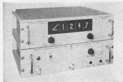
Type 524A2 digital phase meter offers phase angle in degrees directly represented in four digits. Phase reading is independent of the ratio of signal amplitude. Analog or digital output is available for external recorder or programable systems.
