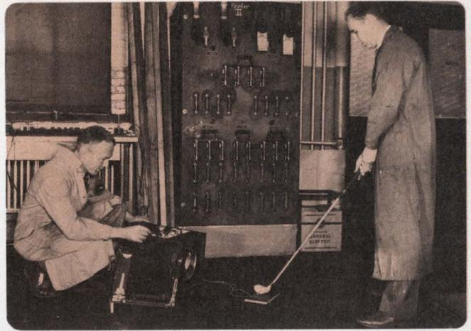
**Harold E. Edgerton** is about to take a swing at a golf ball. A unique electronic circuit for high-speed photography called the stroboscope is operated by Kenneth Germeshausen to record the event. Edgerton is credited with invention of the device. Germeshausen aided in the design. (Photo courtesy of Massachusetts Institute of Technology.)
