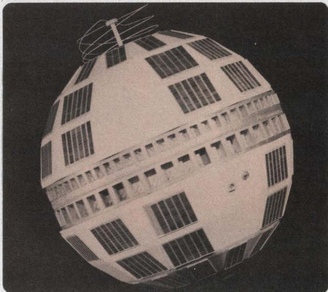
**Telstar, the first active communications satellite**, was also the first privately owned satellite. Its construction and launch in 1962 were financed by AT&T. The 170-lb satellite marked the first international attempt to transmit TV pictures and sound by use of an active-repeater station in space.
