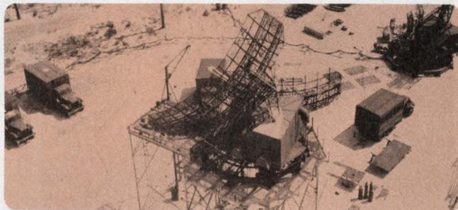
The V-beam radar was one of the most important developments to come out of MIT's Radiation Laboratory during World War II. It was considered the first practical do-everything radar. (Photo courtesy of Massachusetts Institute of Technology.)
