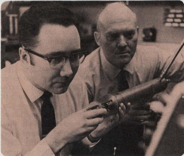
A new microwave source, the Impatt diode, was discovered in the mid 1960s by Bernard LeLoach (left) and Ralph Johnston (right), along with Barry Cohen. The three Bell Labs researchers made the diode emit microwaves by pulsing it until an avalanche of carriers had been produced internally.
