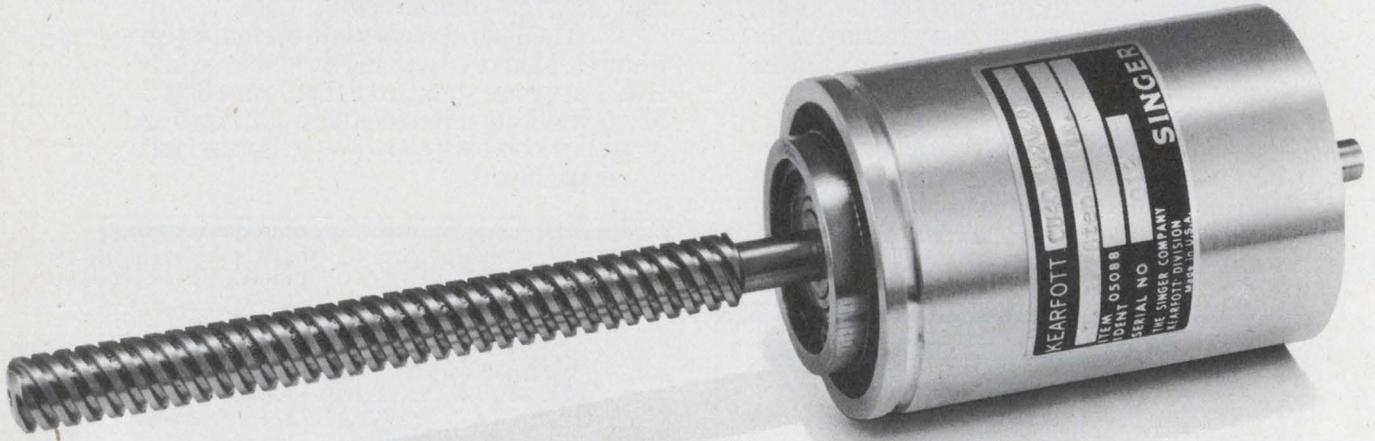
The motor shown above was specially designed with a head positioning lead screw for a "floppy-disc" computer memory.
