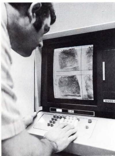
Fingerprints via satellite are displayed on a television screen by "instant replay." The fingerprints were transmitted from Sacramento, California to Tallahassee, Florida by NASA's Hughes ATS-1 satellite and recorded on an Ampex videofile system.
