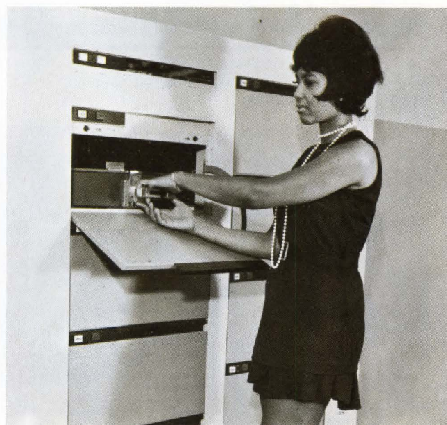
MASSTAPE Pacs are loaded into drive stations that contain the access logic drives.
